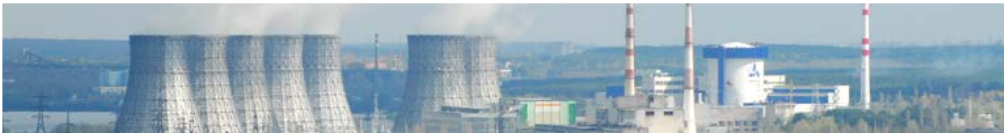
Novovoronezh Nuclear Power Plant
